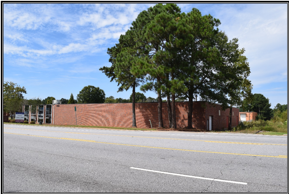
Photo 4: View of 4538 Hugh Howell Road, constructed in 1966, facing northwest.
