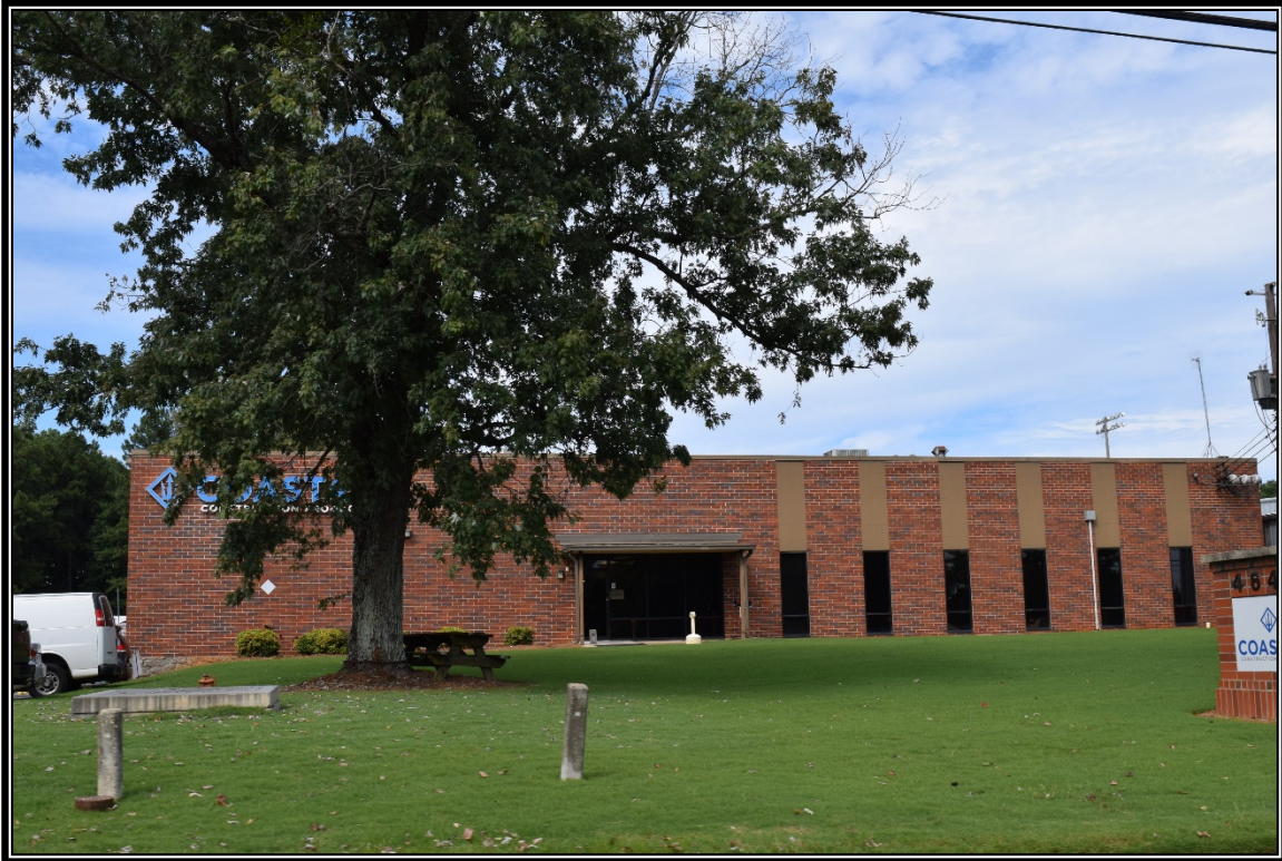
Photo 27: View of 4559 Granite Drive, constructed in 1973, facing south.
