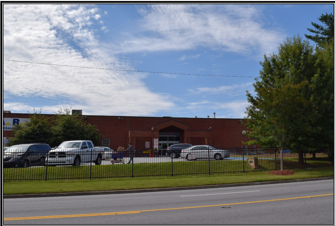
Photo 18: View of 2158 Mountain Industrial Blvd, constructed in 1967, facing west.
