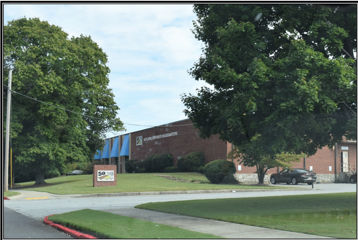
Photo 26: View of 4675 Granite Drive, constructed in 1966, facing southeast.
