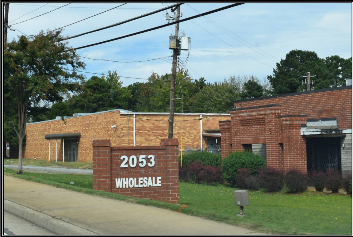
Photo 13: View of 2053 Mountain Industrial Blvd, constructed in 1963, and 2063 Mountain Industrial, constructed in 1964, facing northeast.
