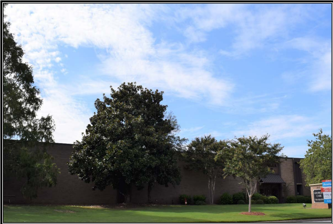
Photo 14: View of 2050 Mountain Industrial Blvd, constructed in 1971, facing west.
