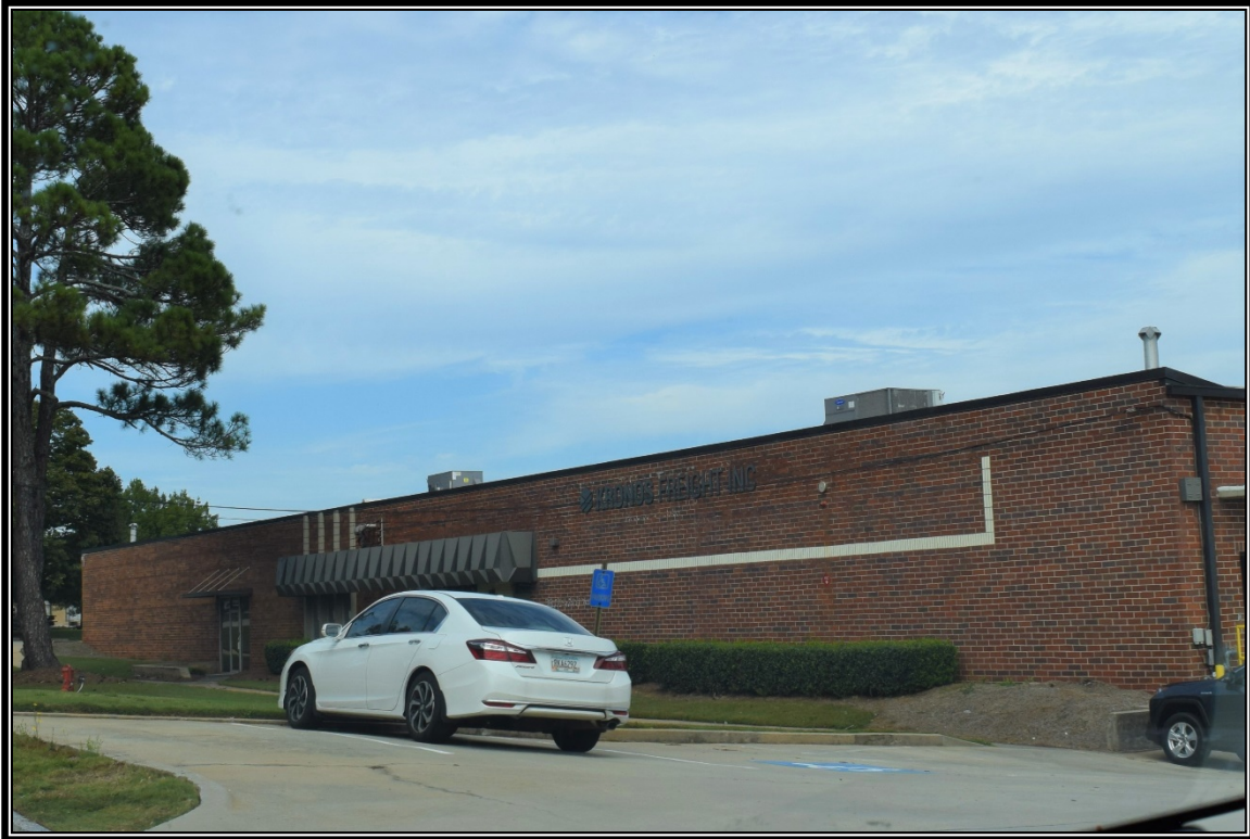
Photo 7: View of 2101 Tucker Industrial Road, constructed in 1963, facing northeast.
