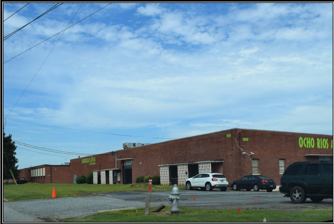
Photo 11: View of 1989 Tucker Industrial Road, constructed in 1964, facing northeast.
