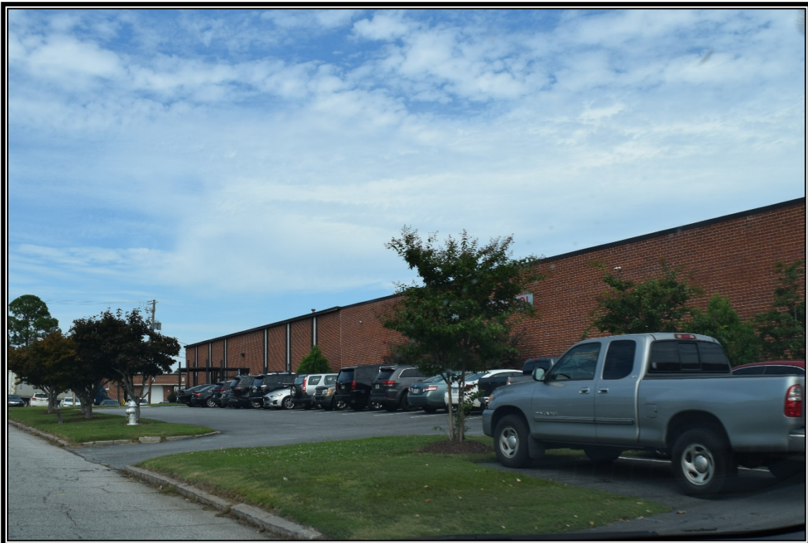
Photo 8: View of 2075 Tucker Industrial Road, constructed in 1964, facing northeast.
