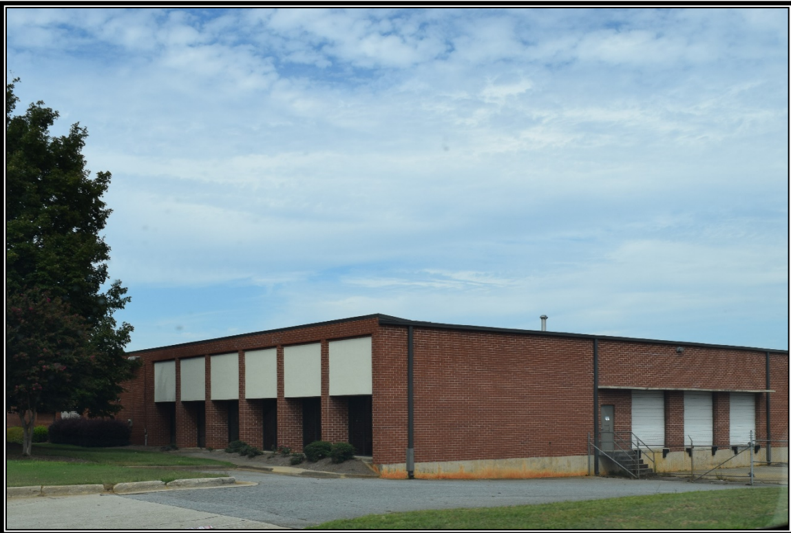
Photo 10: View of 2029 Tucker Industrial Road, constructed in 1972, facing northeast.
