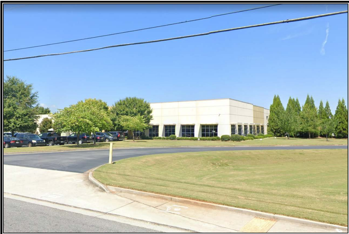
Photo 12: View of 2008 Mountain Industrial Blvd, constructed in 1964, facing north. Photo from Google Street View.
