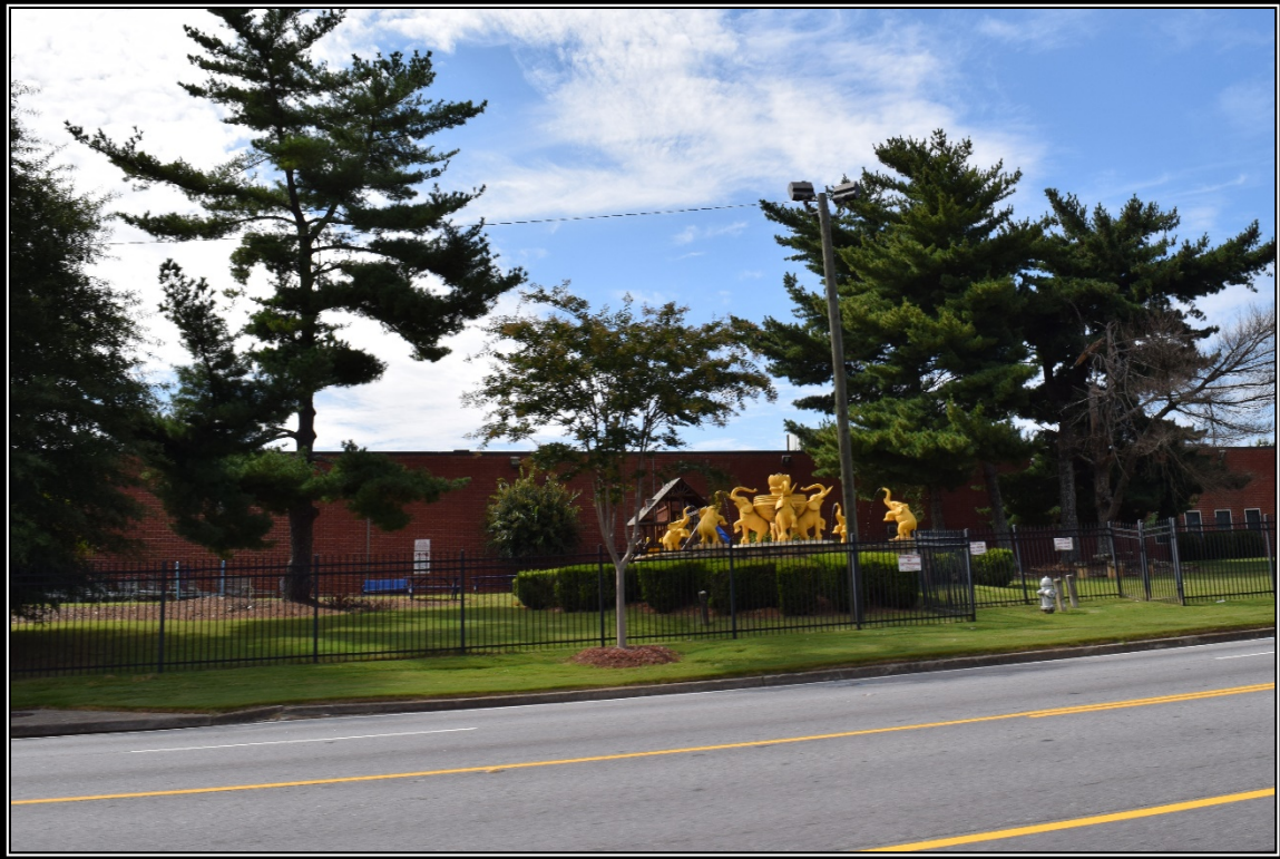
Photo 19: View of 2158 Mountain Industrial Blvd, constructed in 1967, facing northwest.
