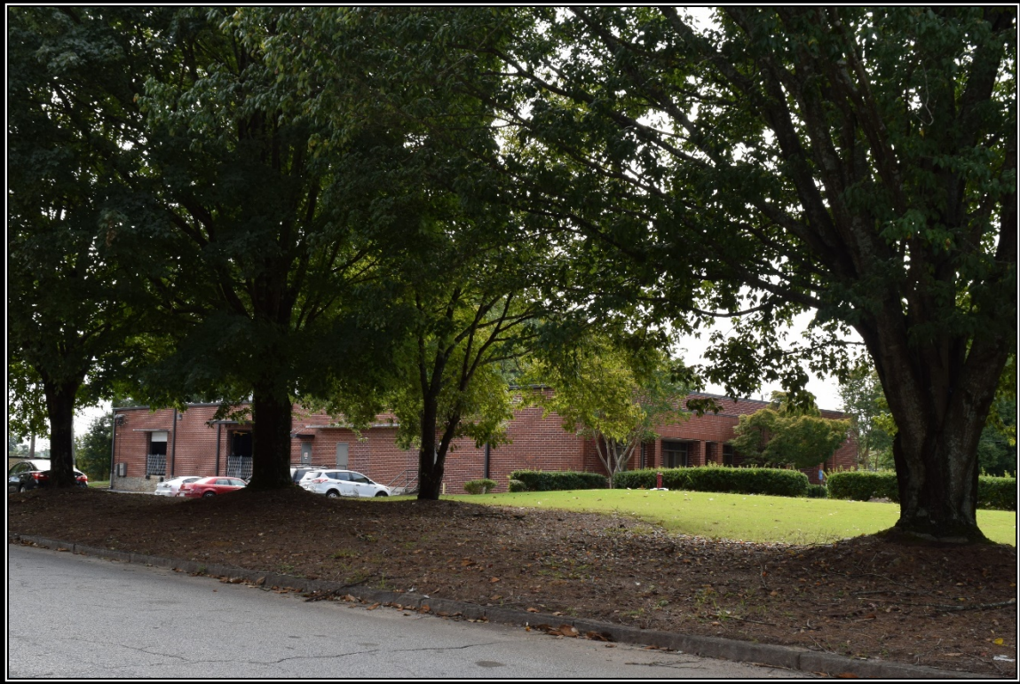
Photo 21: View of 4745 Hugh Howell Road, constructed in 1965, facing southwest.
