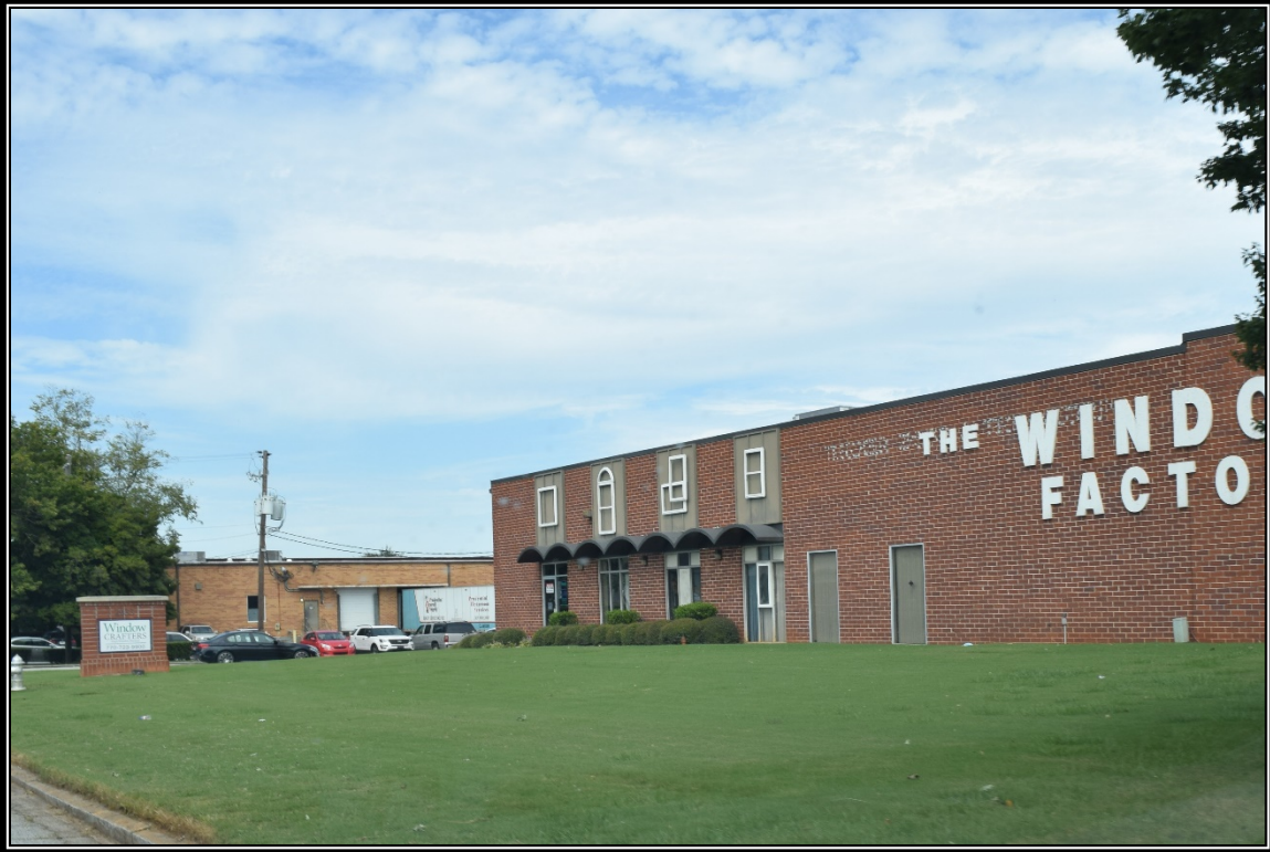
Photo 9: View of 2033 Tucker Industrial Road and 2055 Tucker Industrial Road, both constructed in 1964, facing northeast.
